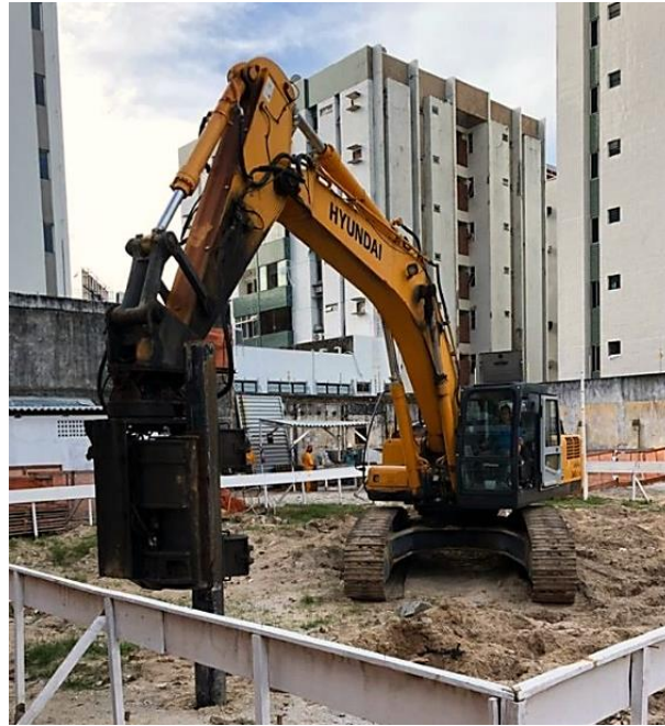
Figure 4: Insertion of the tube using terra-probe method without material introduction [17]
