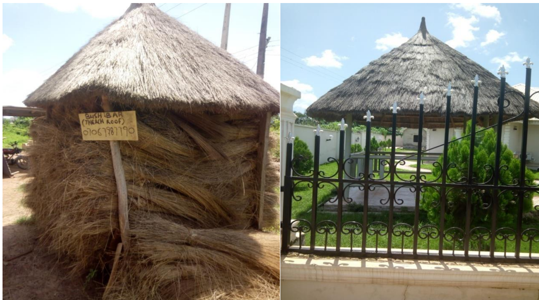
Figure 3: Thatches in stock with roof in place
