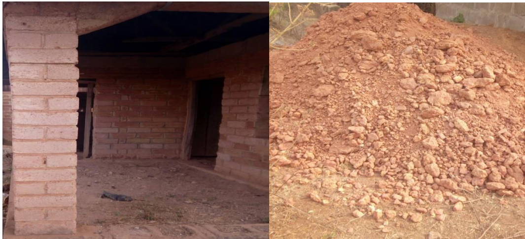
Figure 2: Earth brick column and the materials that used to made it.
