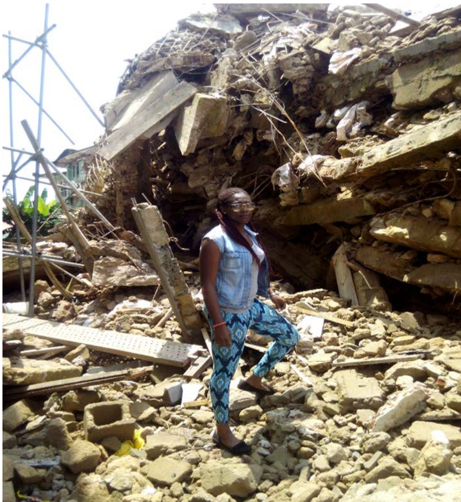
PLATE 2: COLLAPSED 5 STOREY BUILDING AT NO. 10 UDI OBANYE STREET FEGGE ONITSHA ANAMBRA STATE, NIGERIA.
