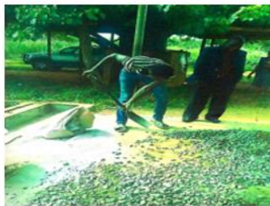
Figure 1: Batching process of Aggregates .
