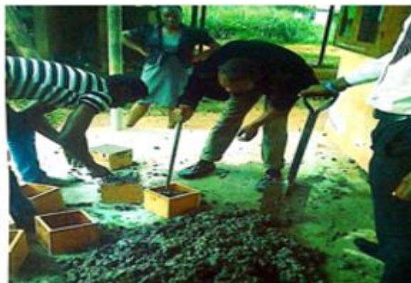
Figure 2: Casting and Compaction of fresh concrete cubes.
