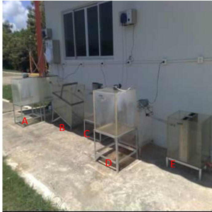
Figure 2: Sequence of the Pilot Station: A) Chemical Precipitation; B) Decanting; C) Ammonia stripping; D) pH correction; E) Reactive Barrier; F) Mixing Box for Lime and Water; G) Mixing Box for Acid and Water.
