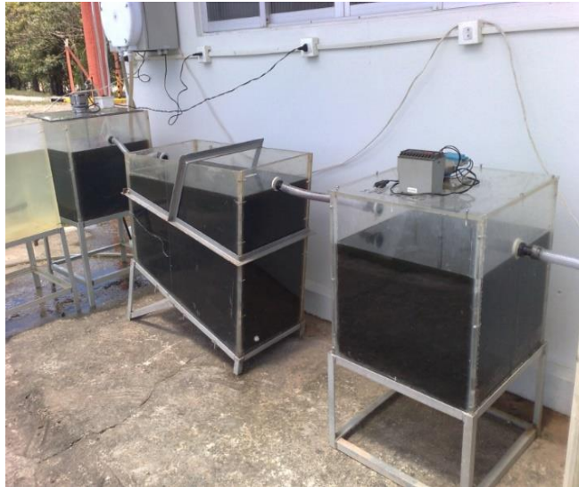
Figure 3: Start-up of the System in Pilot Scale.
