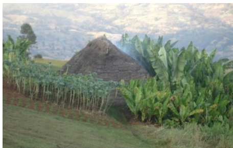
Figure -26- exterior view of Gamo vernacular houses
