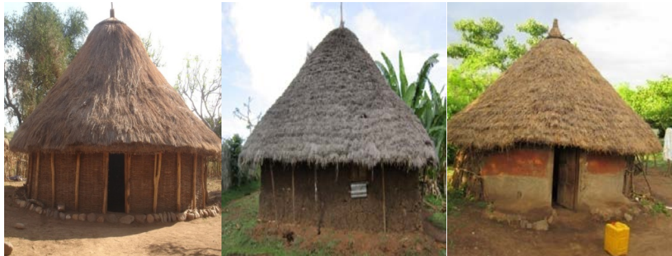
Figure-4.A- Exterior view of "Kaara" type house from; Kamba malo, Ezo, shara communities respectively / This type of design is communal in both lowlands and high lands of Gamo woredas/
