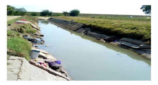
Figure 3: Deterioration of canal Lining in Kyaukthanbet Canal, Mattaya Township, Saedawgyi Irrigated Area
