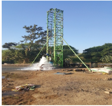
Figure 15: Tube well digging work in Mandalay area
