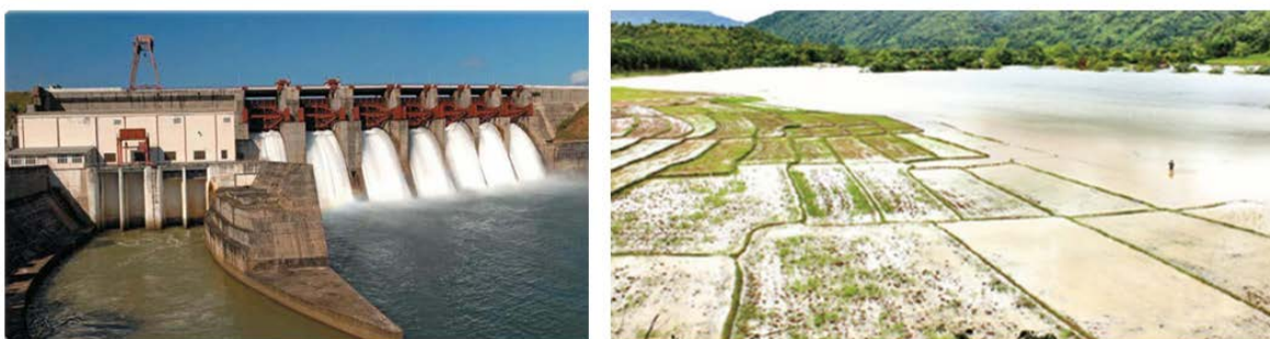
Figure 3: Overflowing from Spill Gates and Flooding of Paddy Fields during the Rainy Season in Sedawgyi Dam
