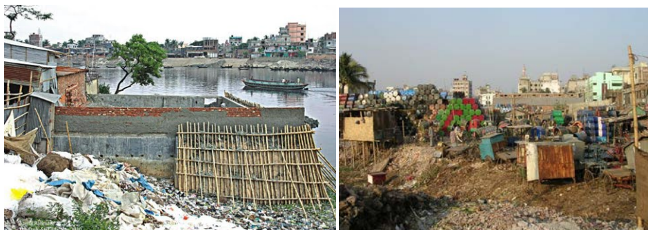
Figure 6: Encroachment (left) and Detrimental Uses (right) of Riverfront.
