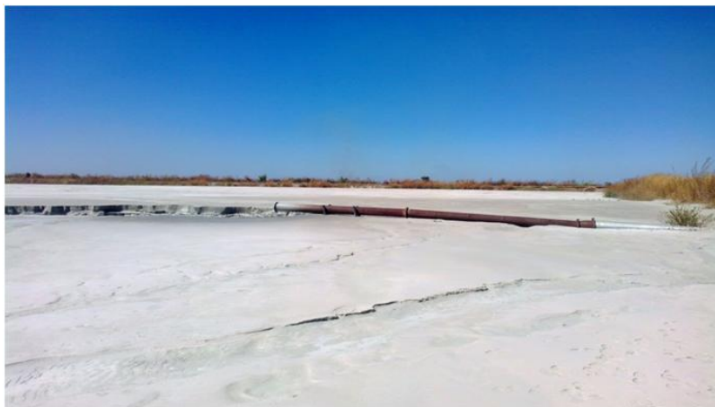
Figure 1: Open-ended Tailings Storage Facility - Musi Dam, Luanshya
