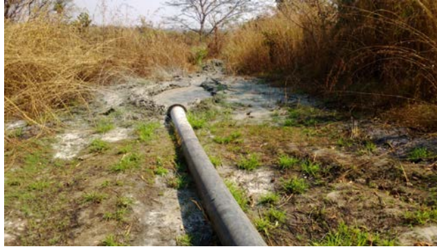
Figure 2: Open-ended Tailings Storage Facility - Musakashi Dam, Chambishi
