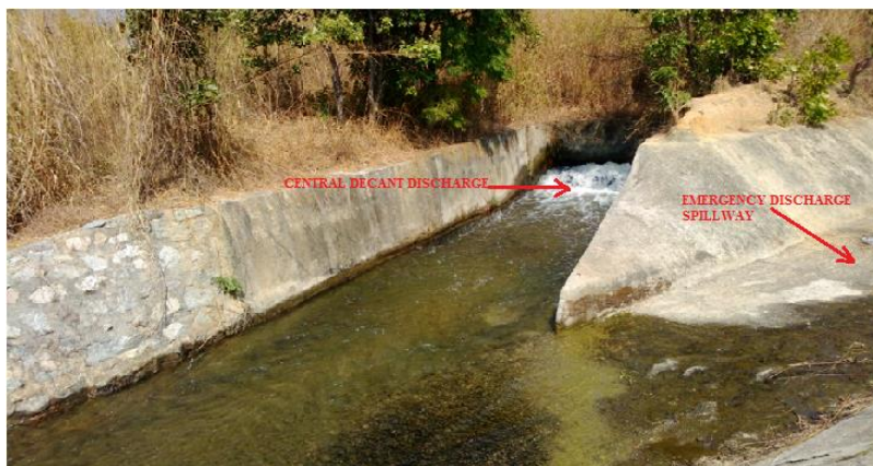
Figure 4: Central Decant Discharge - Musakashi Dam in Chambishi
