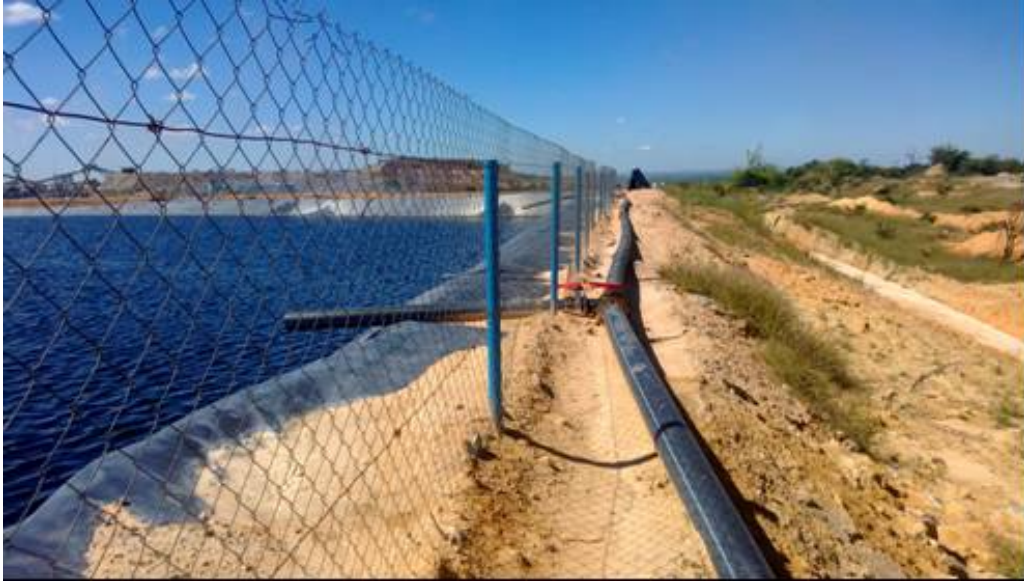
Figure 7: Sino Metals Leach Dam
