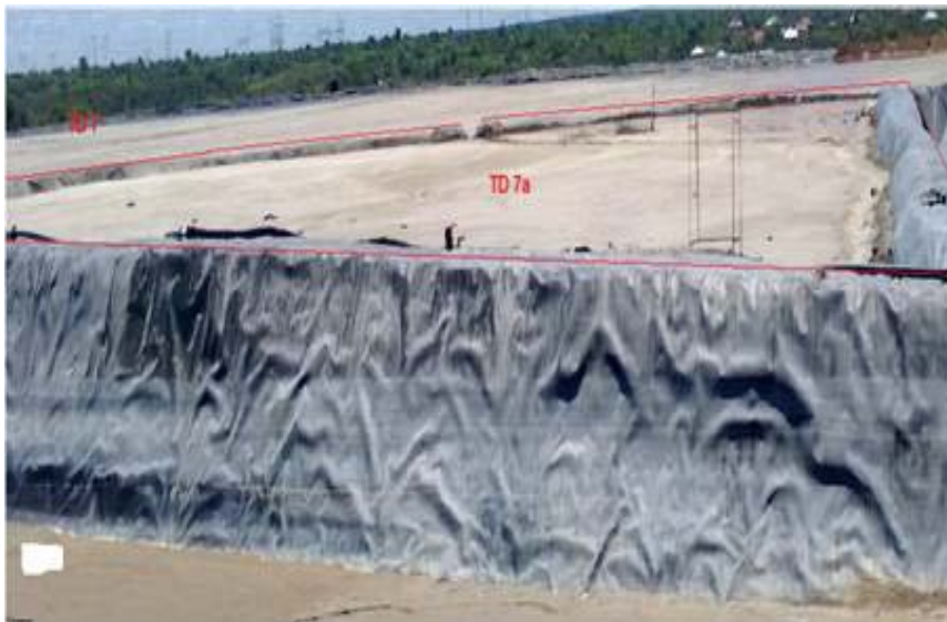
Figure 5: TSF lined with HDPE at Sino Metals Leach Dam
