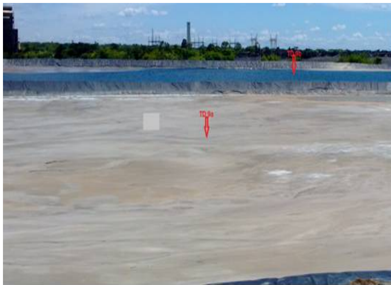
Figure 6: Leach Raffinate clear of solids ready to be pumped back to agitation tanks at Sino Metals Leach Dam
