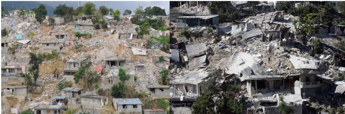
**Figure 6:** buildings built on slopes totally destroyed or damaged during the quake
