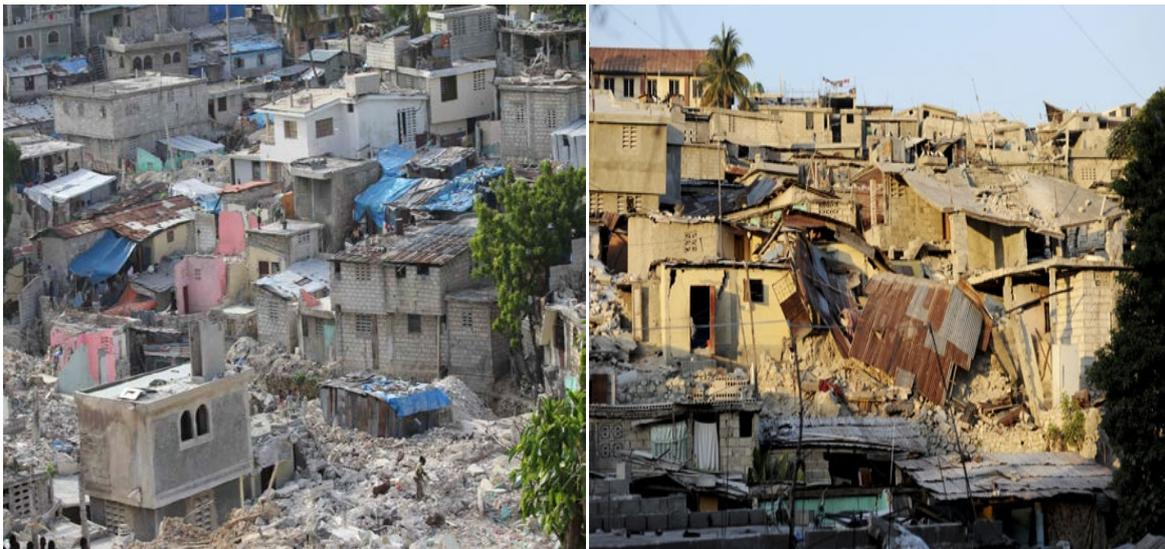
**Figure 8:** non-engineered concrete block walls buildings in Port-au-Prince destroyed by the quake
