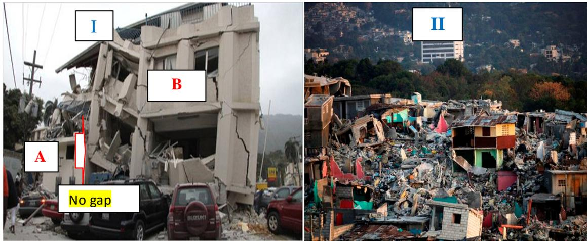
**Figure 10:** Image “I” shows adjacent buildings with no gap and unequal heights and “II” illustrates adjacent buildings built so close that they have been destroyed each other
