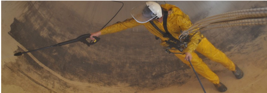
Figure 3: Silo diver using high pressure air jets
