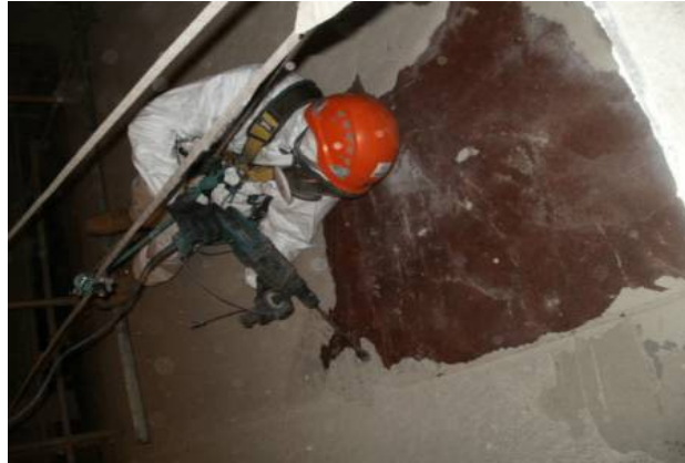
Figure 4: Worker cleaning inside silo using impacting tool
