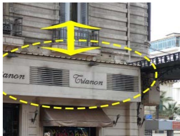
Figure 39: signage compatible with buildings architectural styles.
