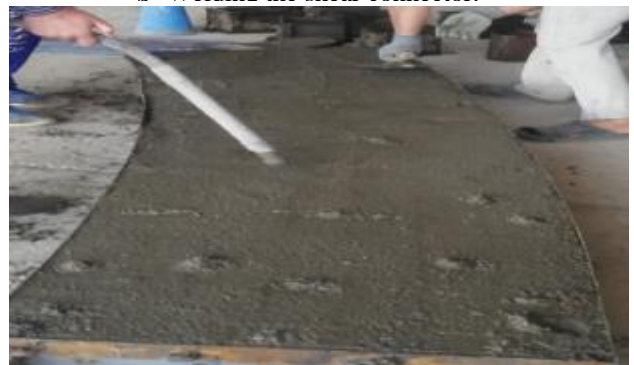
d- Casting the concrete of deck slab
