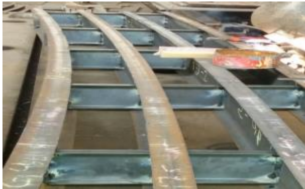
a- Welding Diaphragms with steel curve girders
