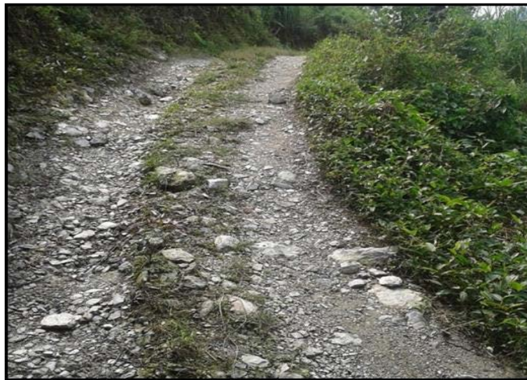
Figure 4: Rut formation in R1
