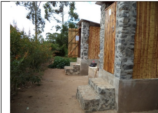
Figure 1: TPS toilet structure
