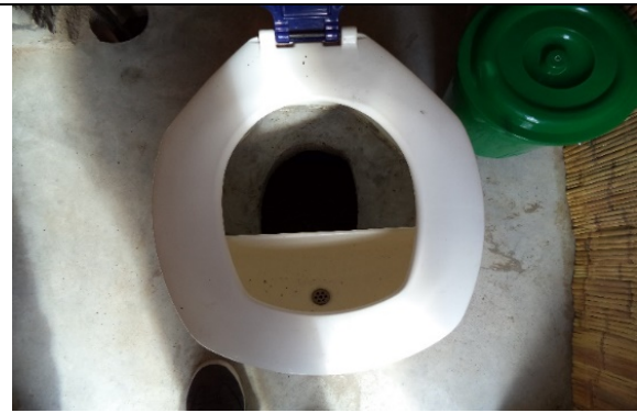
Figure 4: TPS Pedestal inside
