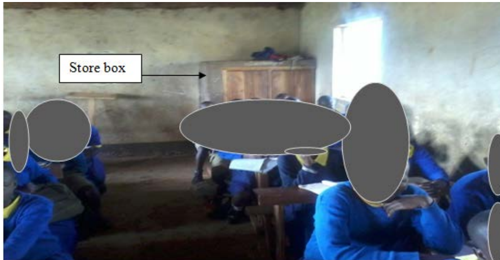
Figure 11: Location of a store box far at the corner with raised doors
