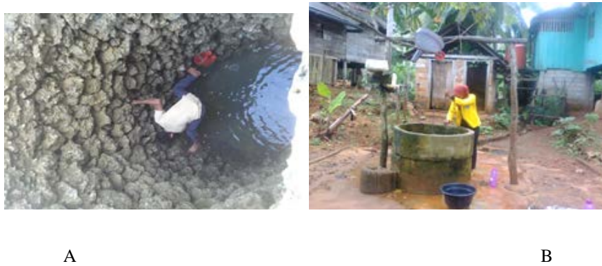
Figure 7: The Dug well construction in Umalaoge Village
