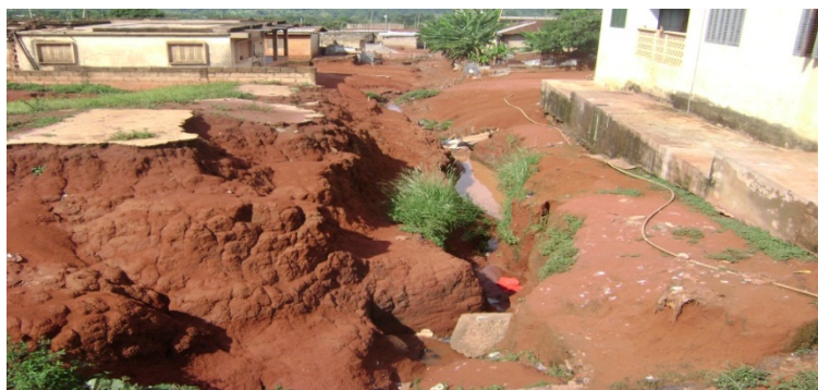
Figure 8: Gully Erosion in the Urban-Subcatchment
