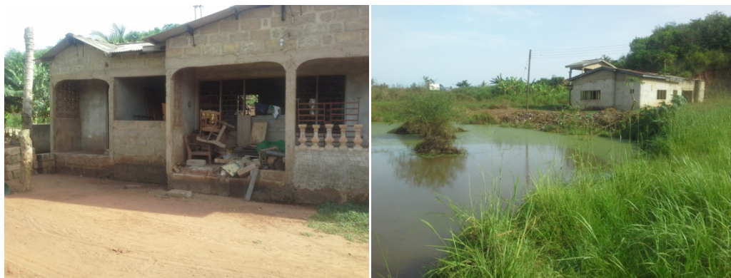
Figure 6: affected residential buildings in Abonko.
