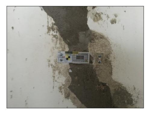
Figure 3: Deformation Markers on the Wall
