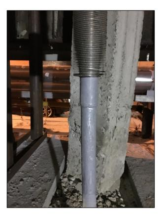
Figure 5: Thermosyphon near Pile
