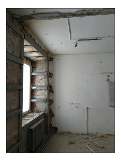
Figure 4: Reinforced Angle Steel Bars Installed for Support
