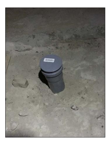
Figure 13: Temperature Monitoring Well Installed on the Studied Site
